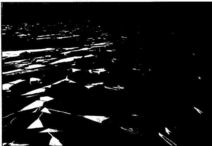
Figure 5. Shatter failure, mechanically attached, nonreinforced membrane.
