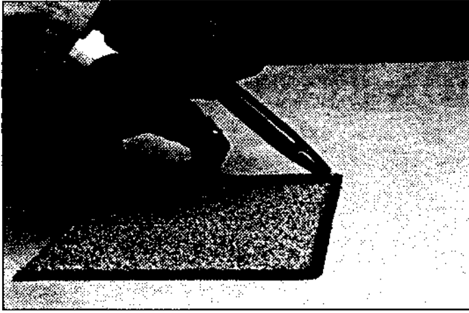
Figure 1. All four edges are herfed diagonally (45-degree angle) to expose the reinforcement.
