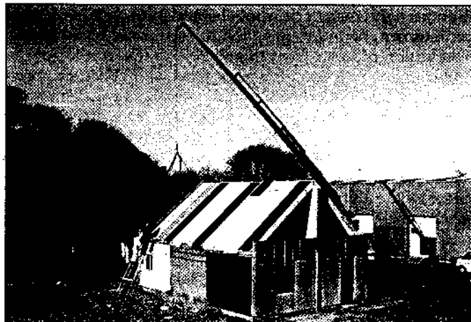
Figure 2. Mounting of roof elements in the test house.
