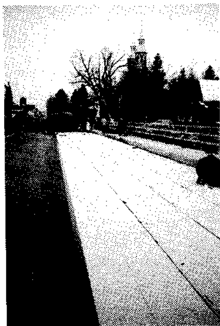
Photo 8: The machine unrolls, welds and presses down on the membrane in a single pass
