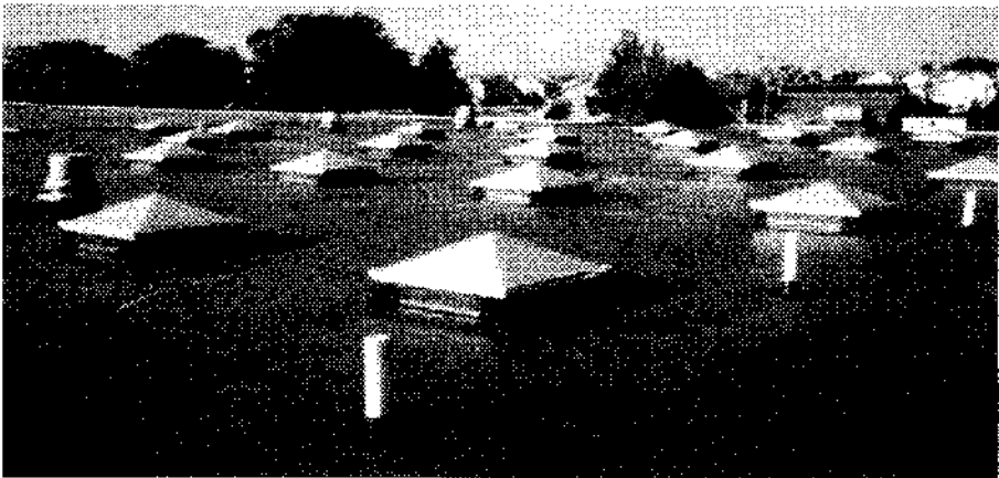
Figure 3: View across skylight field: Designing and successfully installing a tapered insulation system around 36 skylights provided challenges for both designer and contractor. This heavily trafficked area received 60 mil reinforced EPDM for premium performance.
