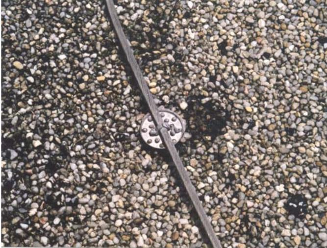
**Figure 8.** *This conductor connector had been adhered in asphalt roof cement to an aggregate-surfaced BUR. Because the cement was applied to loose aggregate, the conductor could be easily moved.*
