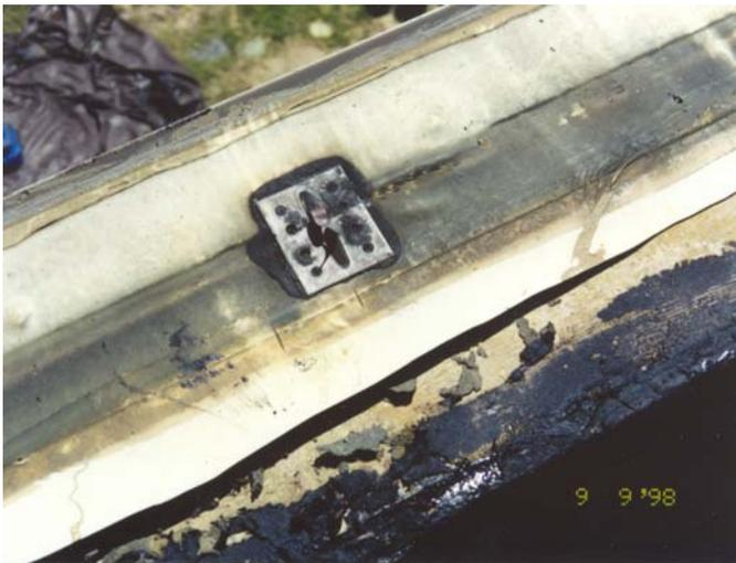
**Figure 15.** In this area, the conductor pulled out from the conductor connector. The connector was adhered to the EPDM membrane.
