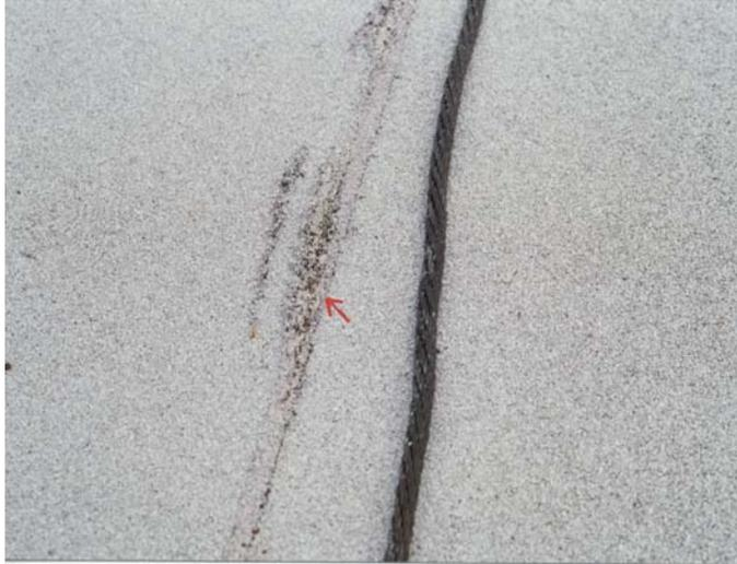
**Figure 5.** *This conductor occurred on a white cap sheet in Florida. The conductor had previously been located to the left where marked by the arrow. At the previous location, the conductor had sunk into the membrane, thereby displacing the bitumen above the reinforcement.*
