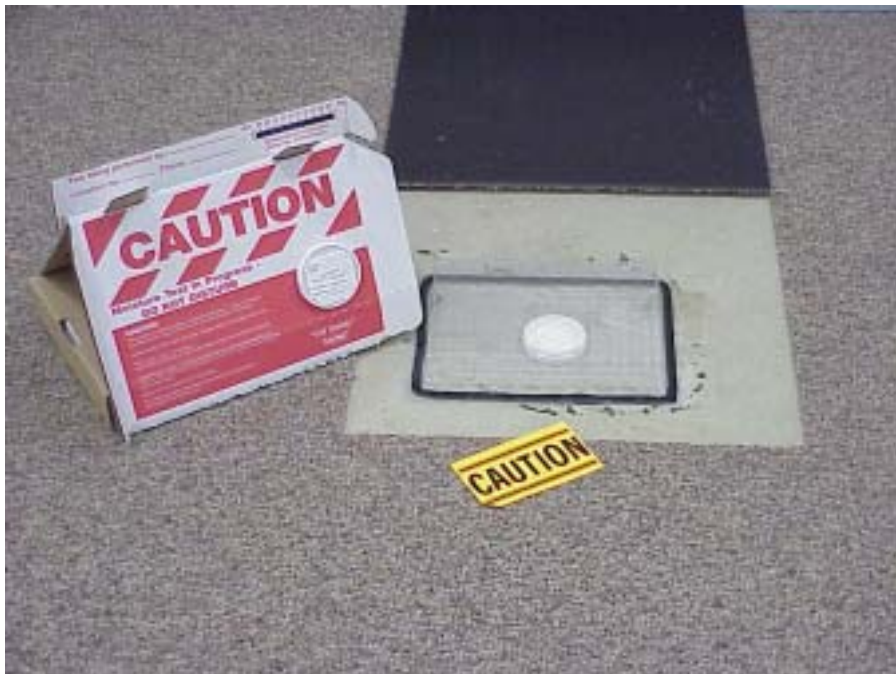
Figure 4 – ASTM F 1869 test being performed for evaluation of carpeting installation on a concrete floor.
