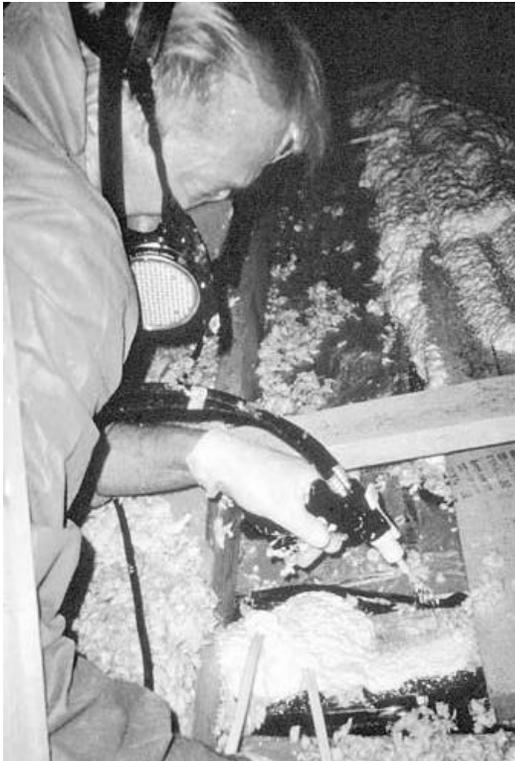
**Photograph 3: The crew lays continuous beads of foam to seal all leaks.**
