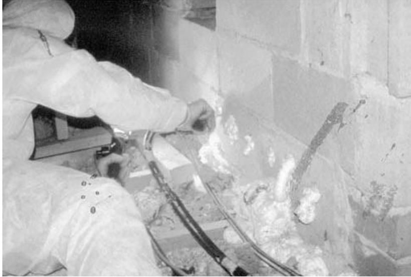
**Photograph 2:** A crew always wears complete safety gear, including disposable Tyvek suits. Here, one crew member is foaming into block cores to stop stack effect within the party wall.
