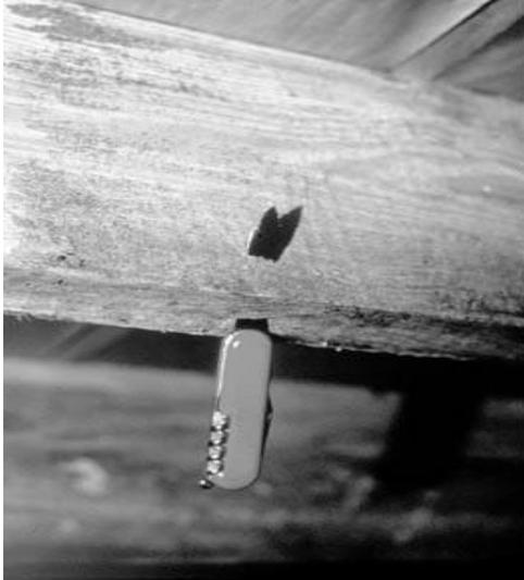
**Photograph 1: Rotting wood is fragile and dangerous, as this pocketknife test shows.**
