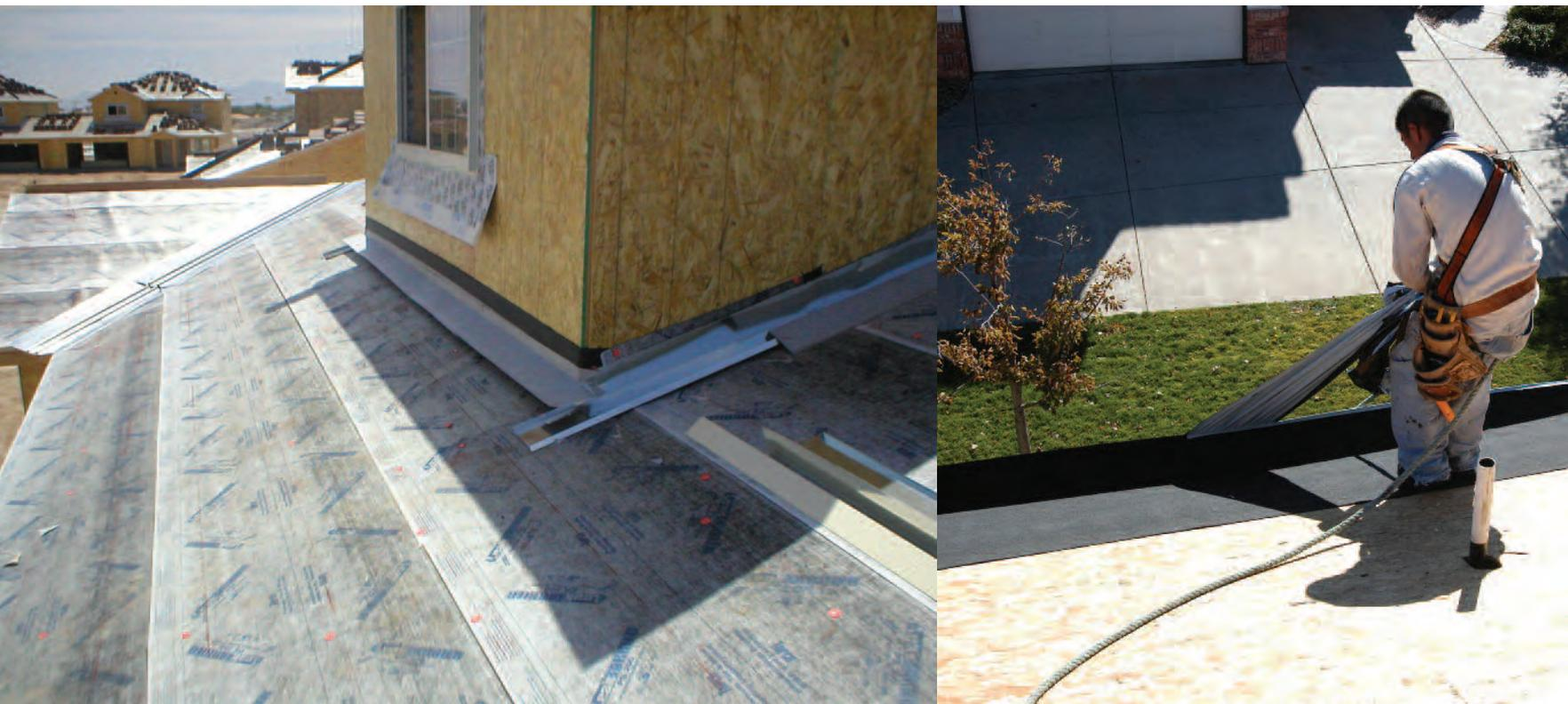
Self-adhering polymer-modified bitumen underlayments provide a weatherproofing layer beneath primary roof coverings, and asphalt-saturated felts are water-shedding.
