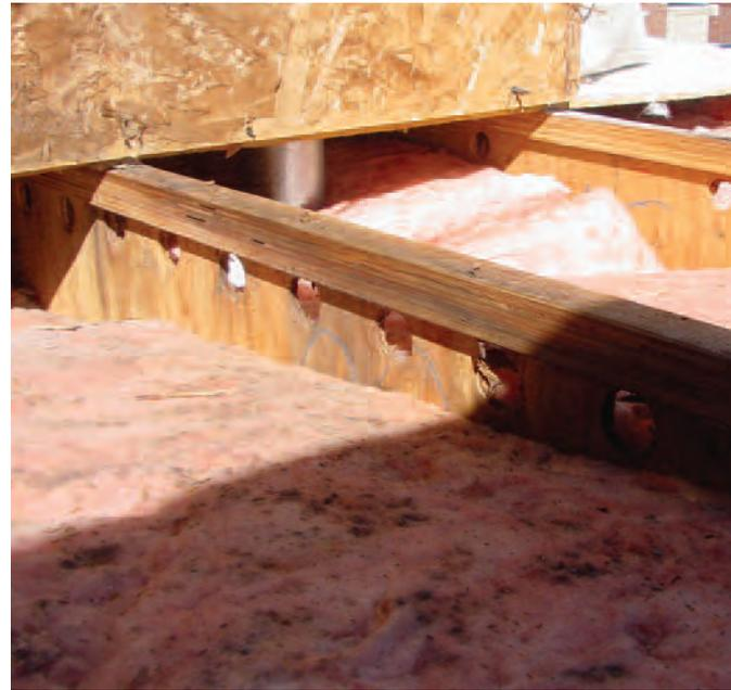
Photo 1: In this low-slope roof assembly, holes are provided in roof framing members in an attempt to provide cross-ventilation.
