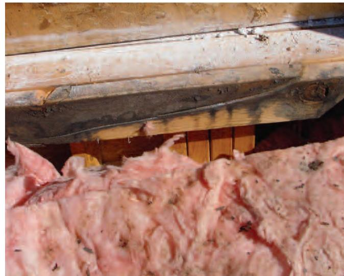
Photo 2: This is a close-up of condensation development on the bottom side of a roof deck in a vented low-slope roof assembly.
