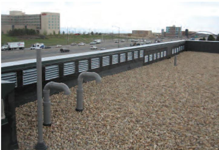
Photo 6: This is an example of prescriptively following IBC 2006’s ventilation ratios. The opposite parapet wall also has the same vent spacing. We calculated that even this quantity was not enough to meet the 1/300 ratio.
