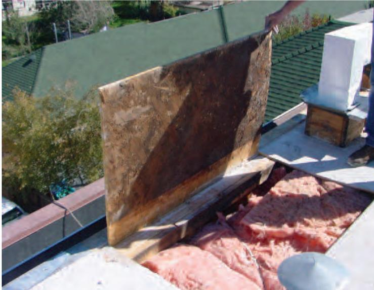
Photo 3: Condensation developed on the underside of roof sheathing in this low-slope roof assembly in a heating climate.
