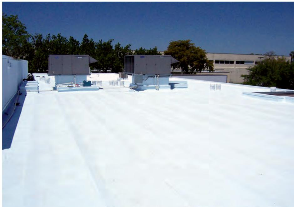
This building's roof system has one coat of a white elastomeric coating. A second coat will hide the substrate, so it will look like a single monolithic white membrane.
