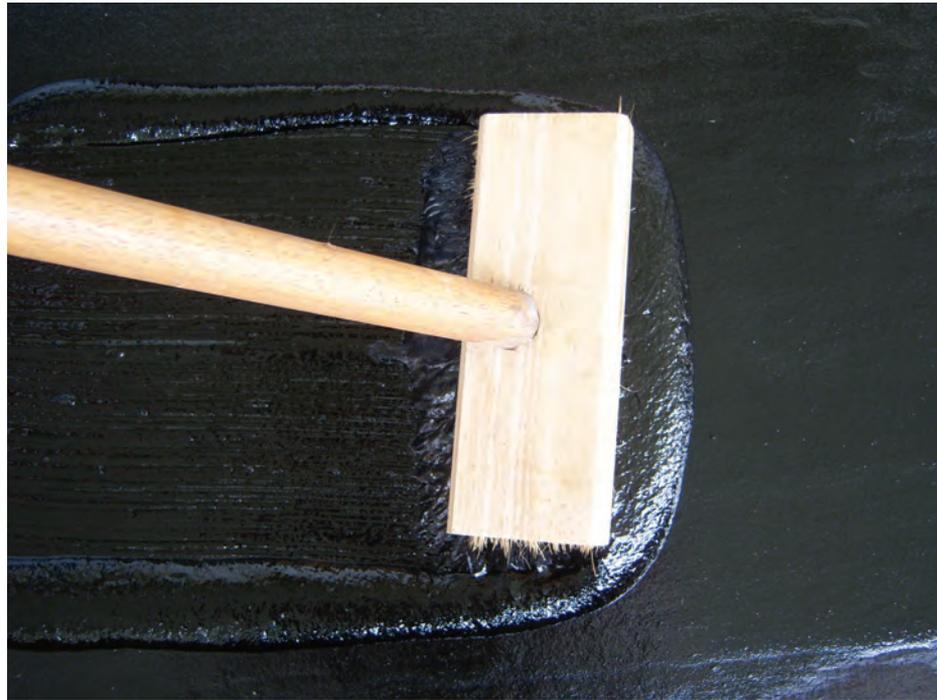
This black fibrated coating is applied with a brush, allowing for thicker application without removing the cellulose fibers.
