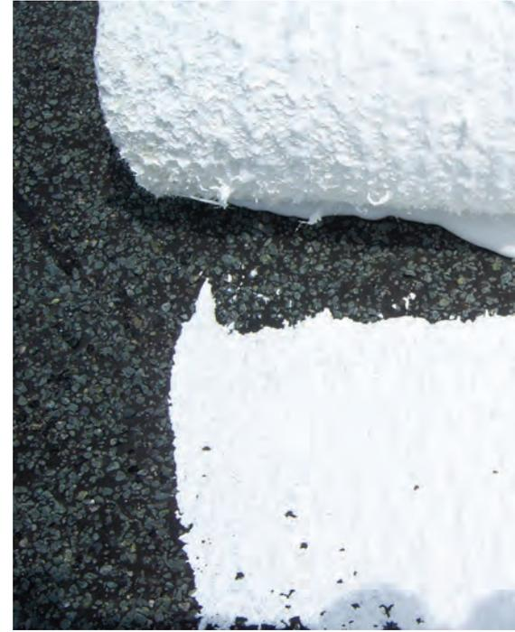
This elastomeric coating is being applied to a surface. The dark surface is visible in the lower left portion of the photo.
