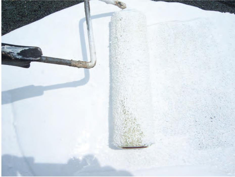
A white elastomeric coating is applied with a roller.
